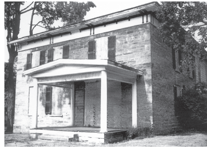
The Jabez Parkhurst house before restoration began
