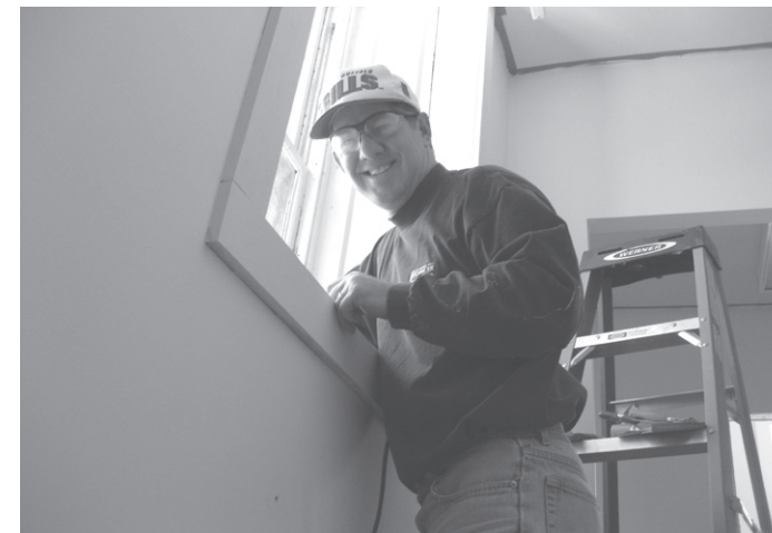
Alan Aguglia dedicated many hours to the woodwork around our windows. Here he is at the top of the stairs on the second floor.
