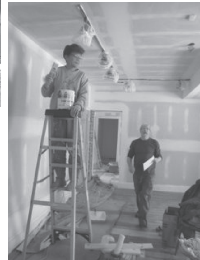
Linda Harwood and David Richardson working on the first floor entrance room.
